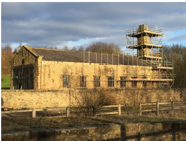
The Soho Engine Shed during essential maintenance works in February (photo: Trevor Horner).
