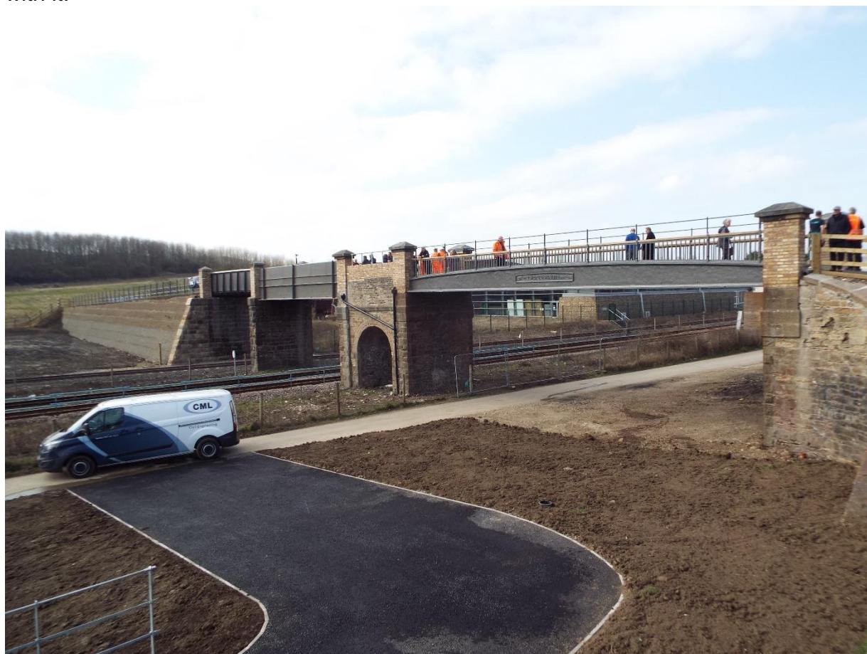
Thickley Bridge – restored, renewed and much more useful! (Photo: Peter Bainbridge)
