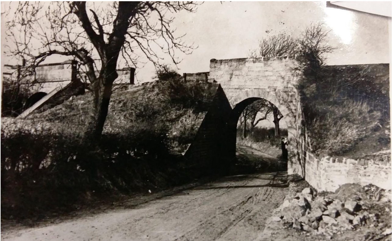
The two S&DR bridges at Brusselton, side by side. The one in front is the simpler road bridge. The one to the left (behind the tree) is the more ornate accommodation bridge, presumably requested by Musgrave. The road bridge was demolished c.1959. The accommodation bridge has fared better having been lovingly restored by Durham County Council and the Brusselton Incline Group (photo courtesy of Jane Hackworth-Young)
