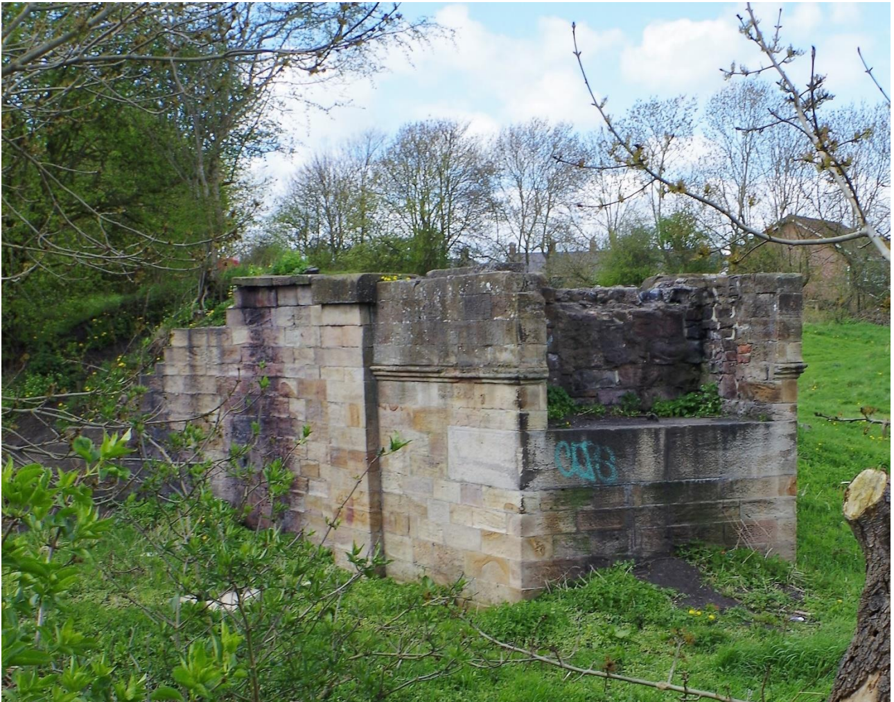
One of the surviving abutments (photo: Niall Hammond)
