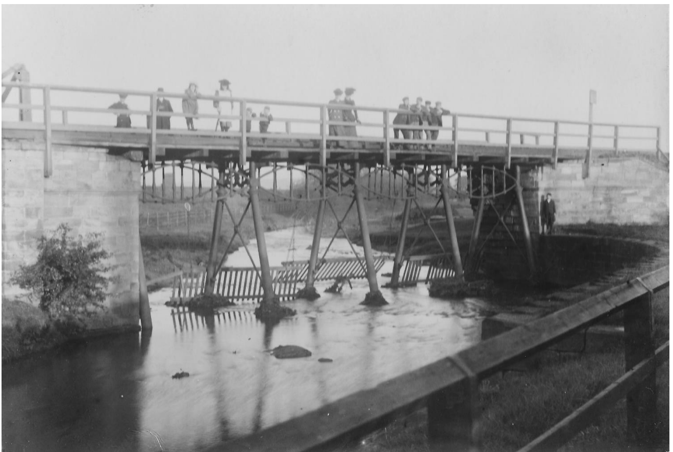
The Gaunless Bridge before 1901
