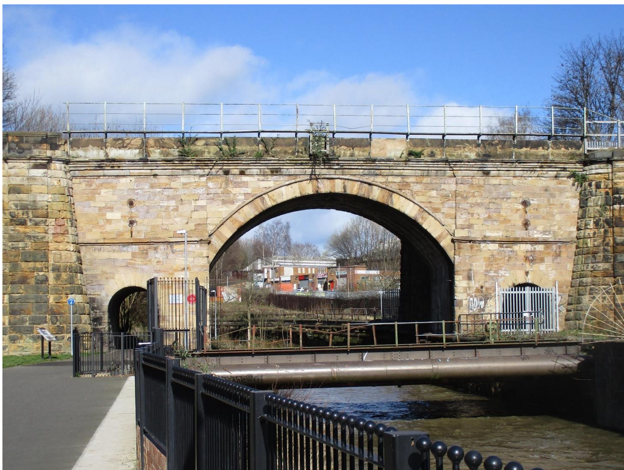
Skerne Bridge: "ingenious centering"
