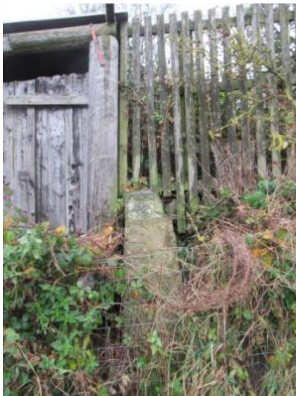
P24 – West Elevation retaining wall
