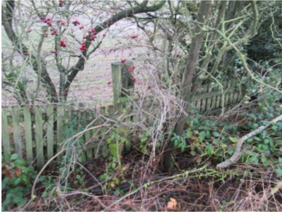
P31 – South Elevation inner boundary timber pale and rail fence
