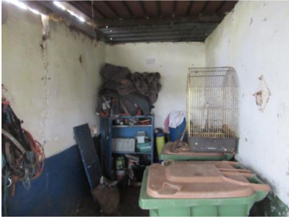
P17 - Interior of the lean-to with inner skin of brickwork built up against the retaining wall
