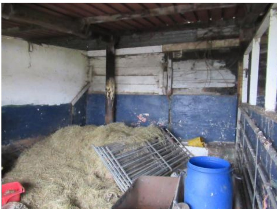
P16 – Interior of the lean-to with inner skin of brickwork built up against the retaining wall
