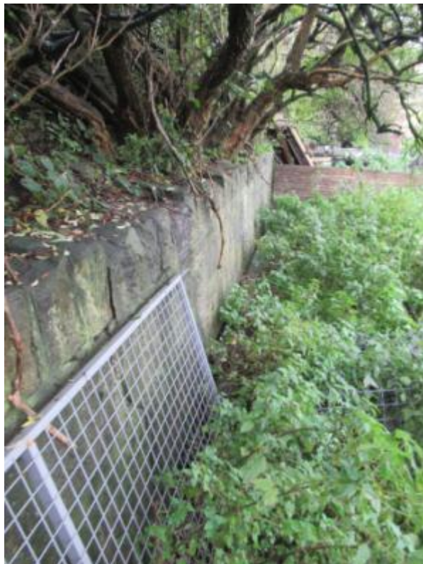
P22 – West Elevation retaining wall reasonably plumb
