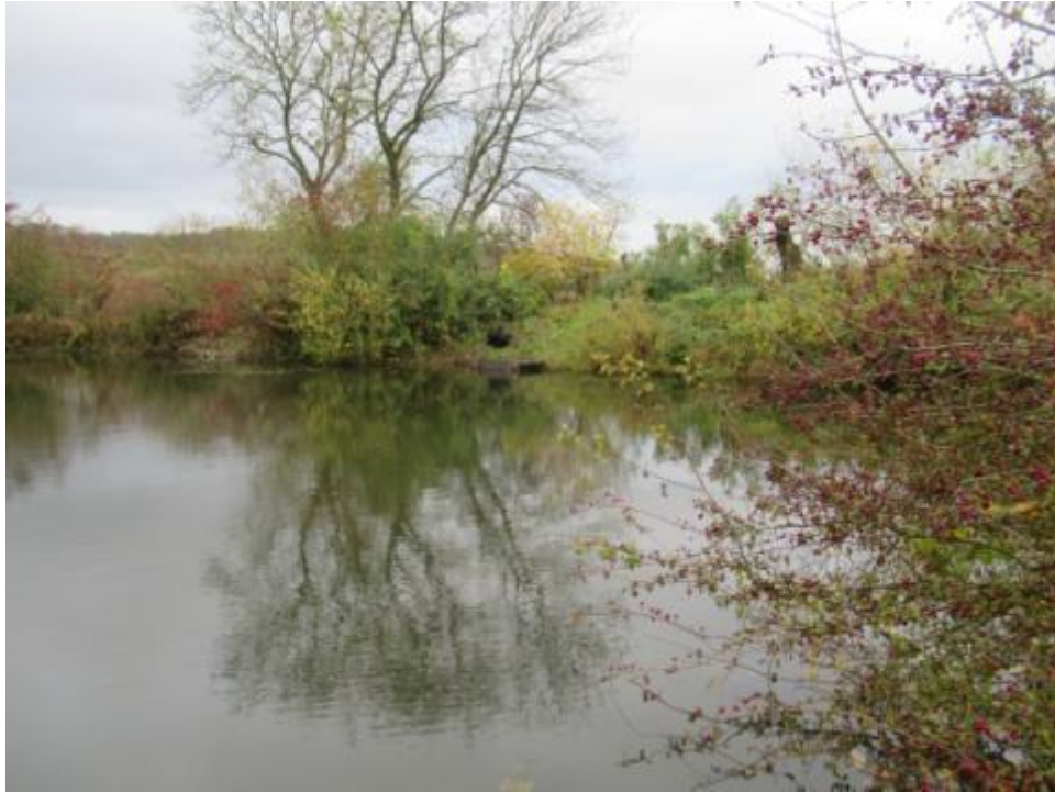
P49 – Reservoir North Embankment
