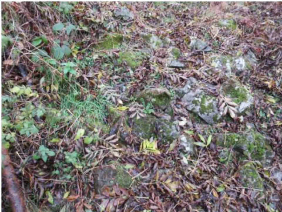
P46 – Reservoir, rubble stone to create Embankment
