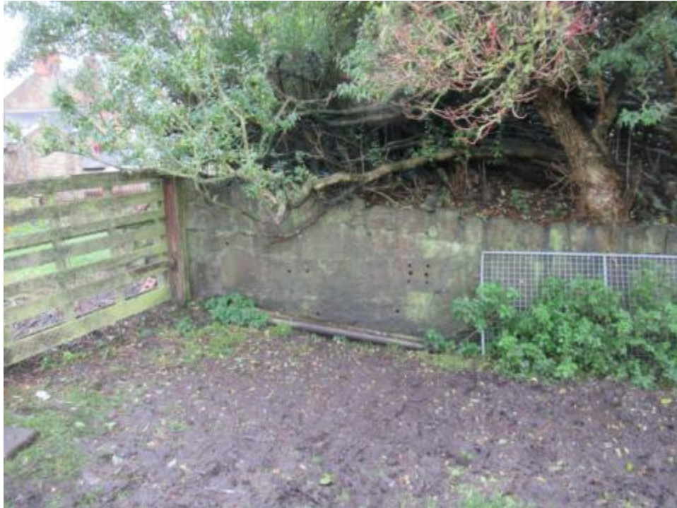
P1 – West Elevation view from the field
