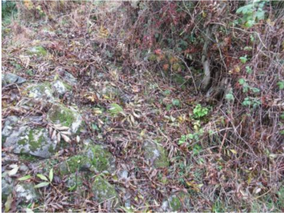
P47 – Reservoir, rubble stone to create Embankment
