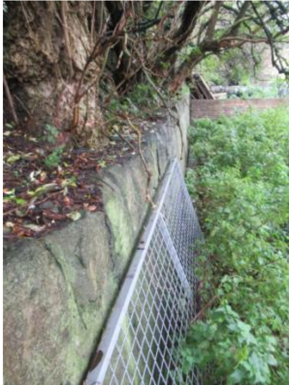
P21 – West Elevation wall reasonably plumb
