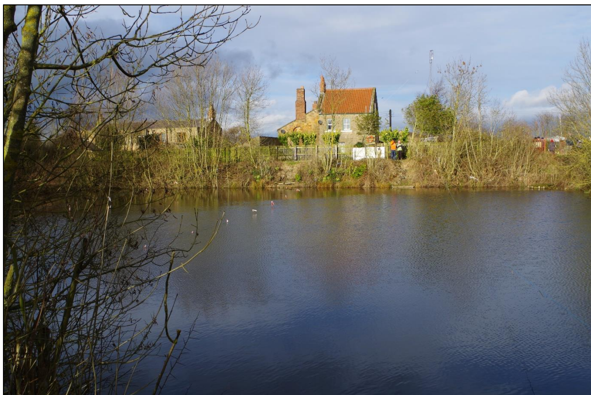
Figure 15. The reservoir looking north towards the Engine House with the roof of the Engineman's house visible to the left.
