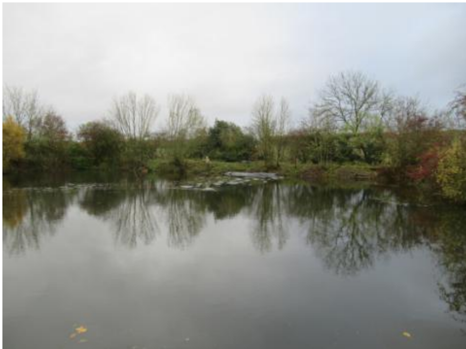
P48 – Reservoir South Embankment
