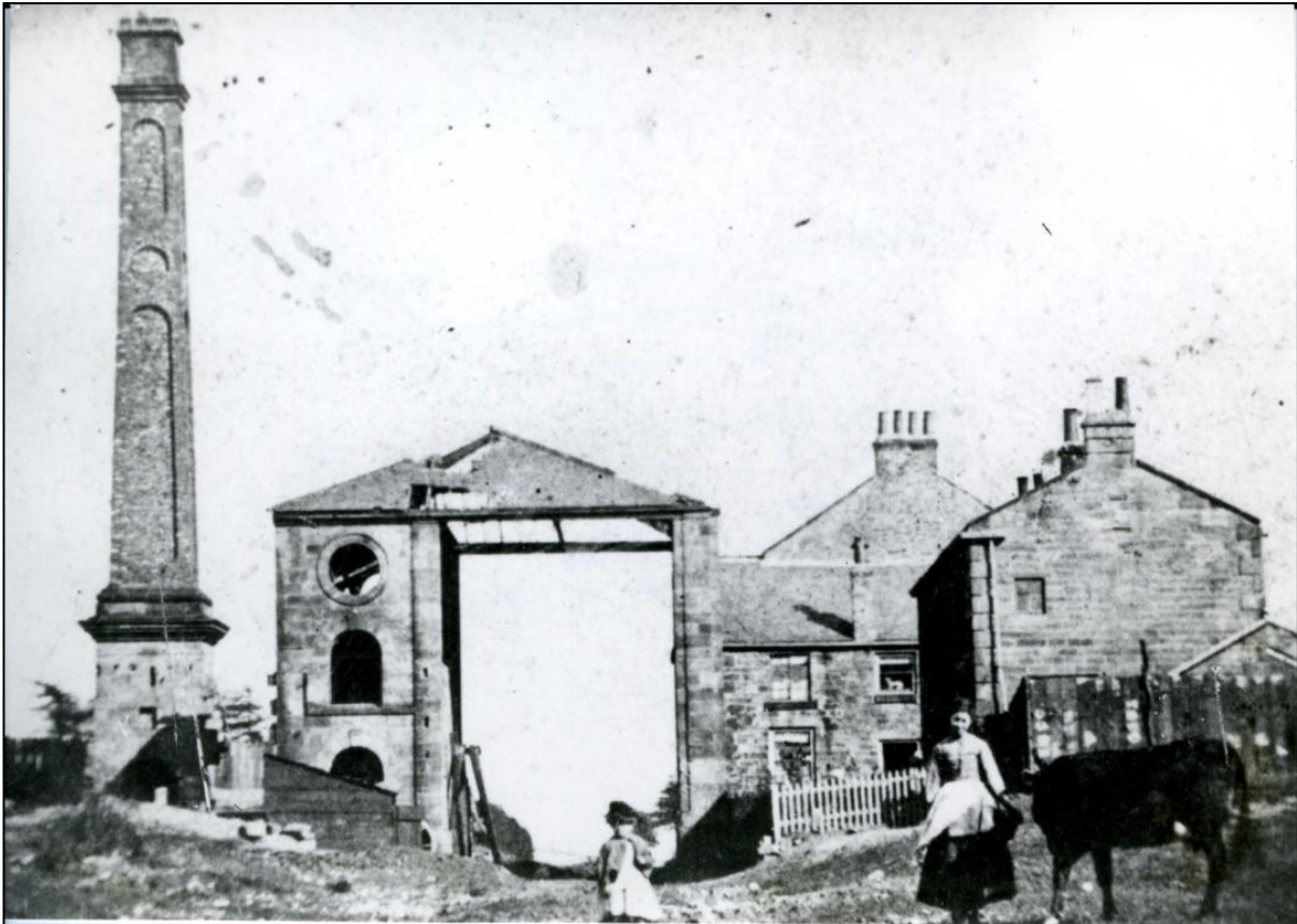
Figure 9. Brusselton Engine House chimney and winding gear house, now demolished (photo courtesy of Jane Hackworth-Young, undated, but possibly c.1880). The large empty building of 1831 held the winding gear which consisted of large drums which sat above the line, powered by the steam engine in the adjacent engine house. This was a replacement of the first Engine House which still survives partially on site today.
