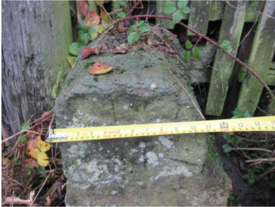
P25 – West Elevation retaining wall top thickness
