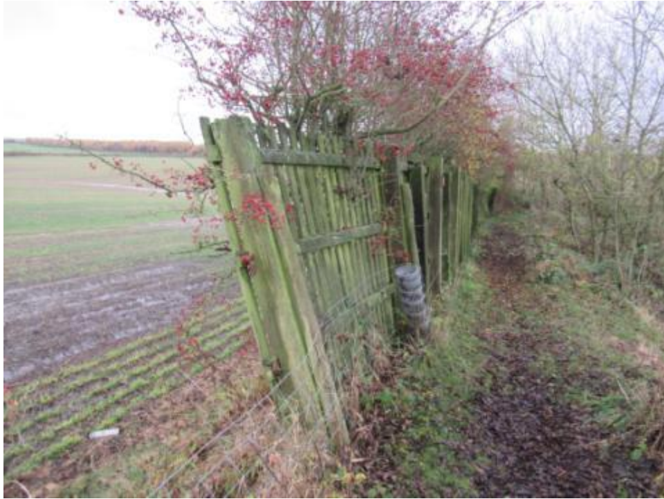
P35 – East Elevation – section missing and collapsed fence
