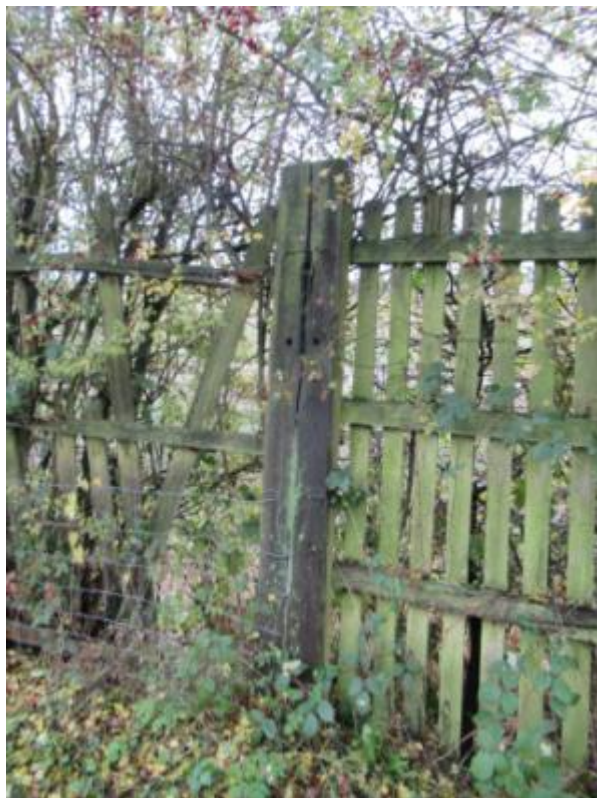
P33 – East elevation railway sleeper for post
