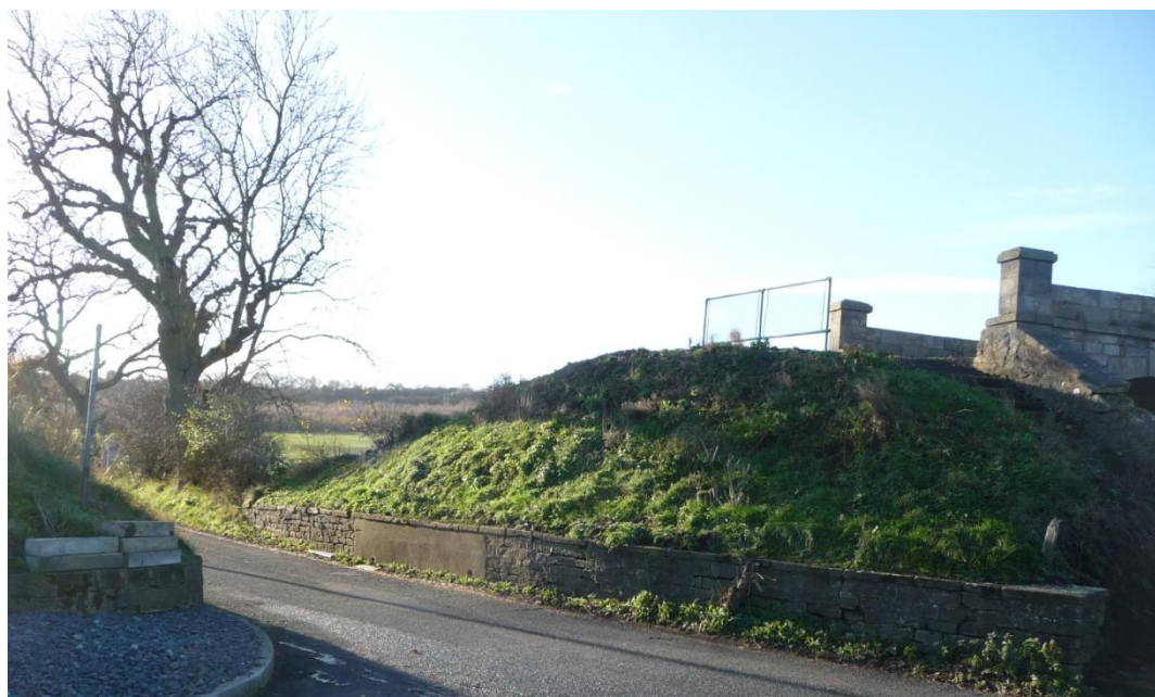
Plate 12. The only visible remains of the road bridge is concrete render over the join where the bridge abutted the embankment on the west side of the road.
