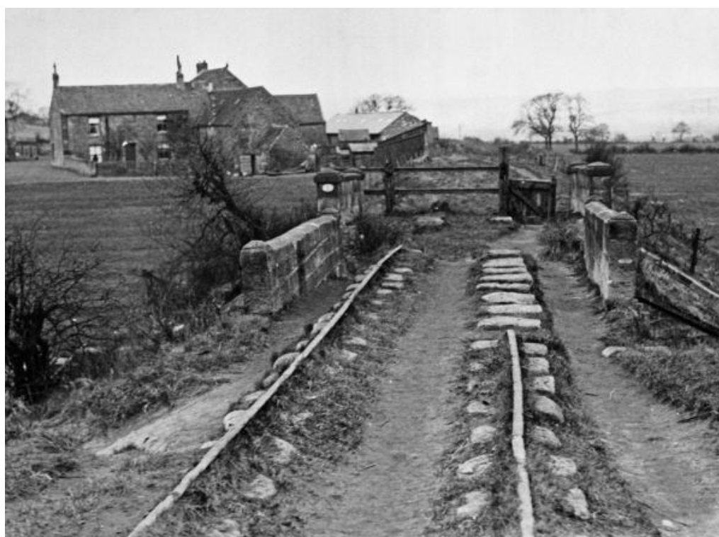
Plate 10. The decking of the road bridge with the accommodation bridge beyond. Both have metal plaques on them numbering them. (Photo undated but possibly 1925, courtesy of Trevor Horner)
