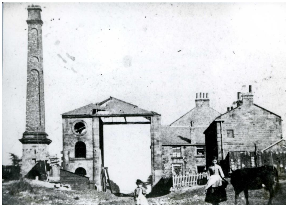
Plate 3. Brusselton Engine House, now demolished (photo courtesy of the Ken Hoole Collection, undated, but possibly c.1880). The large empty building of 1831 held the winding gear which consisted of large drums which sat above the line, powered by Hackworth's steam engine adjacent. This was a replacement of the first Engine House which still survives partially on site today
