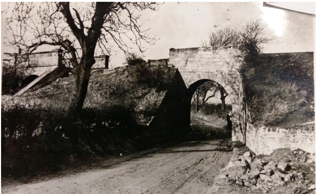
Plate 8. The bridge built to take the S&DR line over Brusselton Lane; the pile of stones suggest that damage or demolition has already occurred to the road bridge which was demolished in the early 1960s to allow for road widening. (photo courtesy of Jane Hackworth Young)
