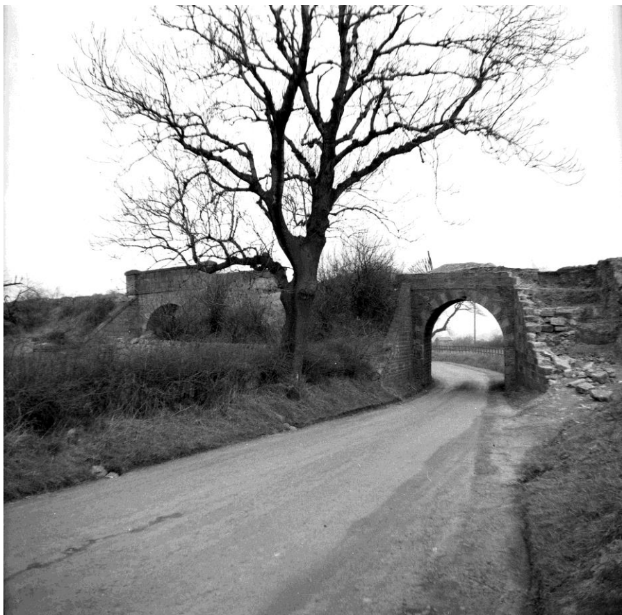
Plate 11. An undated photo of the demolition of the road bridge underway. The exposed structure of the embankment can be seen and it appears to consist of terracing of stone filled with rubble and earth. (Photo: J.W Armstrong/ Armstrong Railway Photographic Trust)
