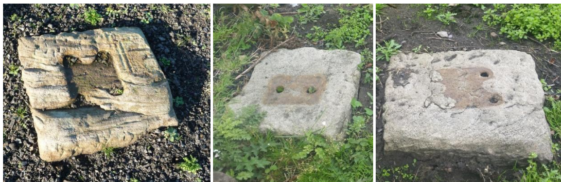
Plate 22. Left: Some sleepers on the incline show markings caused by the rails. Centre: The earliest two hole sleeper. Right: the second phase four hole sleeper to provide greater stability
