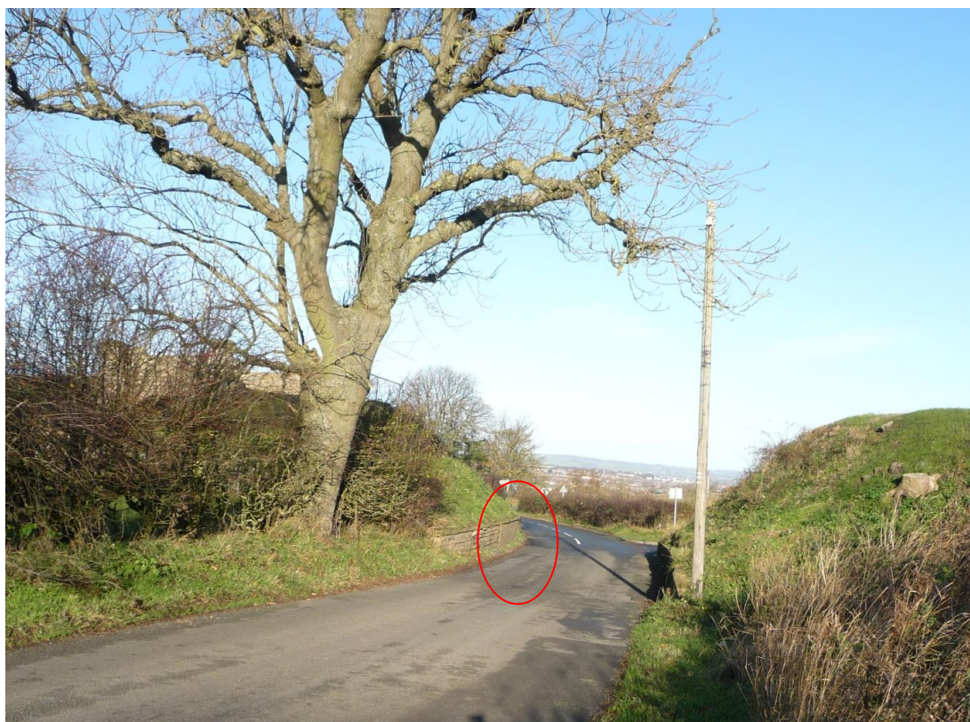
Plate 9. A similar view in 2015. The only evidence of the road bridge is a strip of concrete render on the retaining wall to the left (west)
