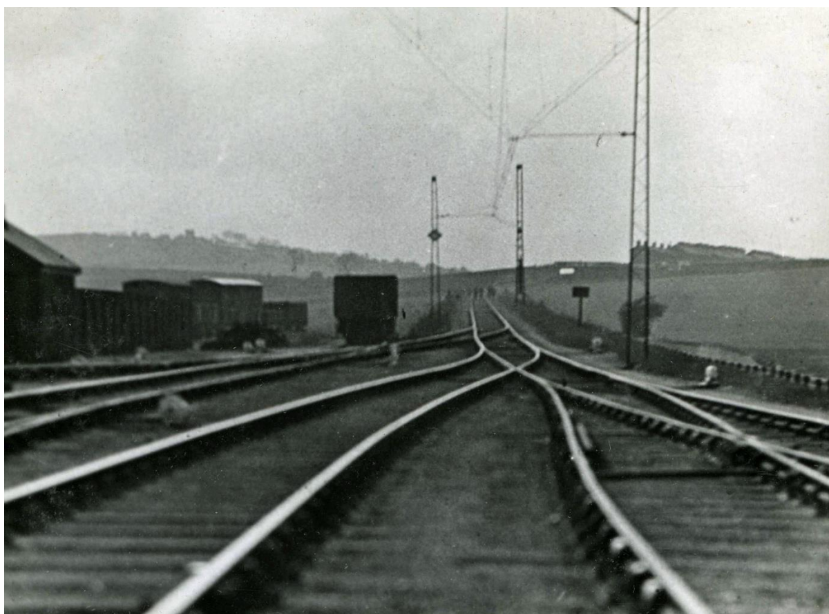
Plate 5. Brusselton Incline east of the Milk Bridge (and so east of Brusselton village and the Accommodation Bridge) with the village and Milk Bridge in the distance. This shows the Brusselton line electrified when it was used as a repair line between the Milk Bridge and Shildon. Photo: from the Ken Hoole Collection at Head of Steam – Darlington Railway Museum
