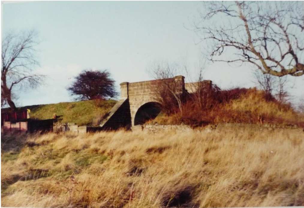
Plate 15. Photo taken from the south looking north of the Accommodation Arch in 1974 at which time, it was described as being in fine condition (John Proud albums).
