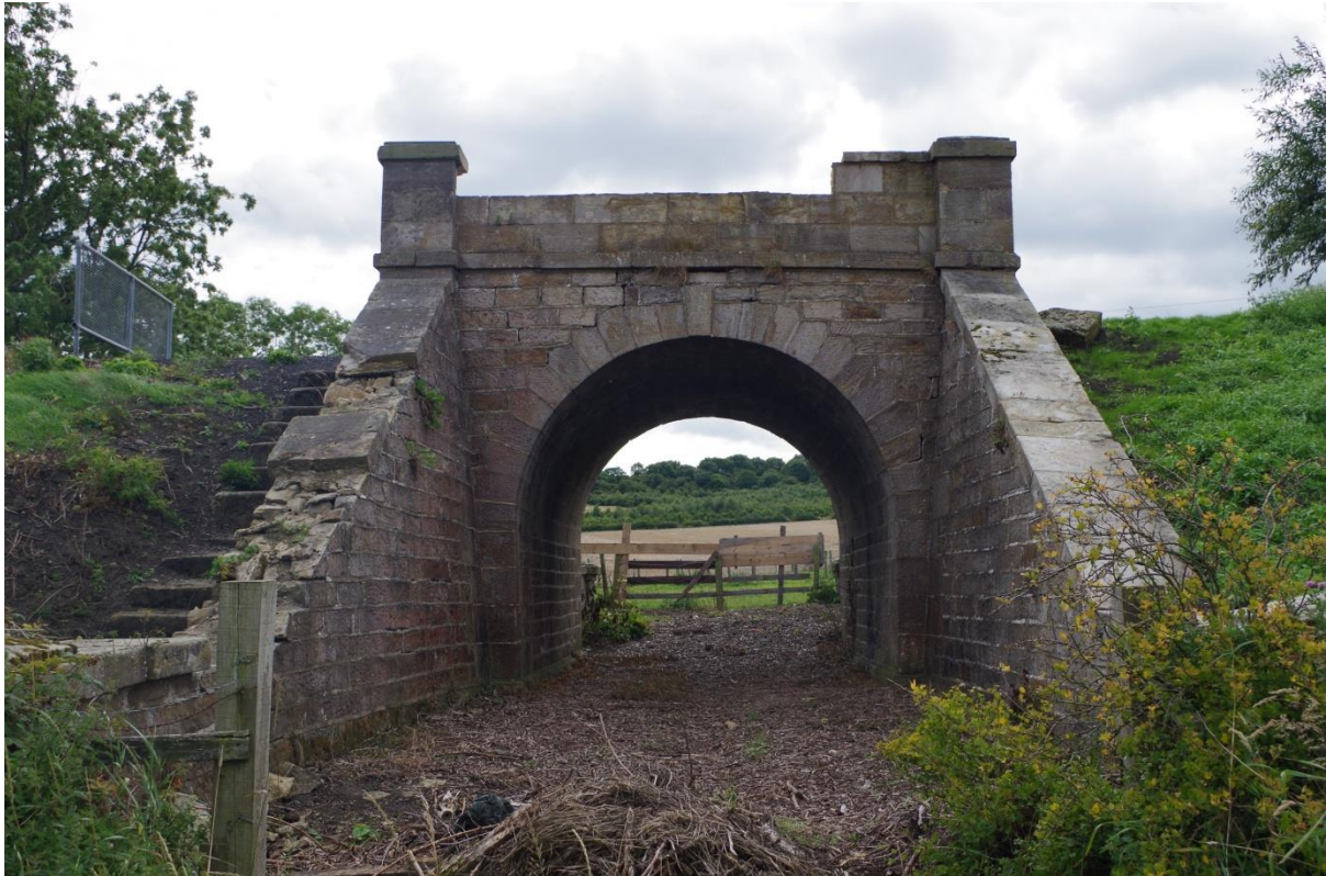
Plate 14. The scheduled accommodation bridge 10m west of Brusselton Lane in 2015
