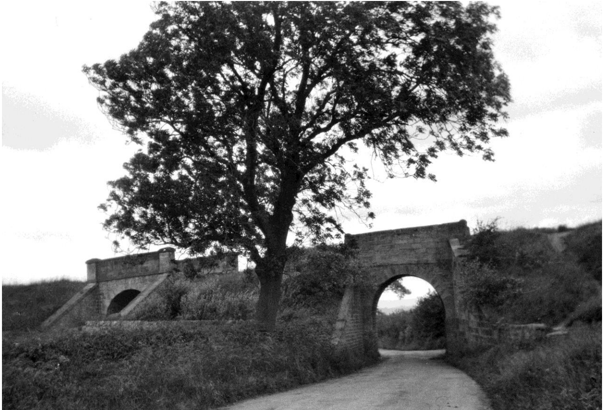
Plate 7. An undated photo showing both the road bridge (right) and the accommodation bridge (left) intact. The surviving Accommodation Bridge appears to be a grander structure with a capped parapet, while the 1825 road bridge is a simple structure with few architectural pretensions (Photo: J.W Armstrong/ Armstrong Railway Photographic Trust)
