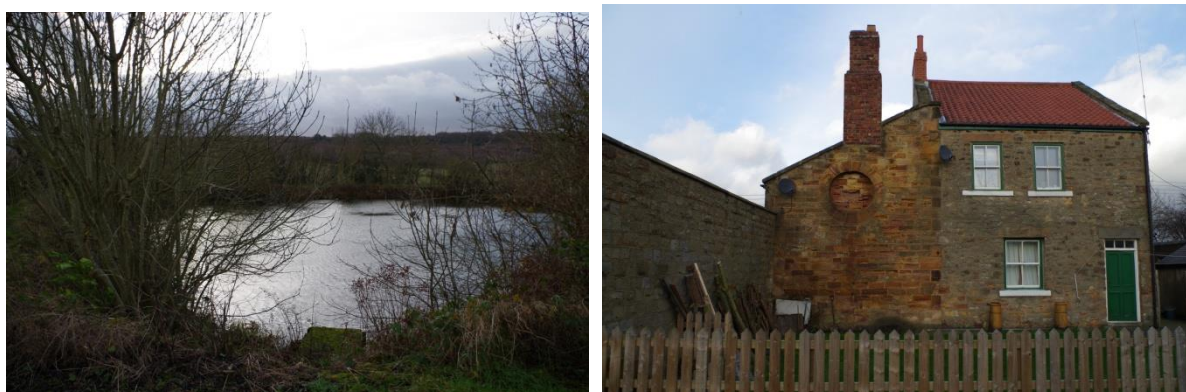
Plate 6. Left: the reservoir that was constructed to feed the engine house. This currently has no legal protection. Right: the engine house
