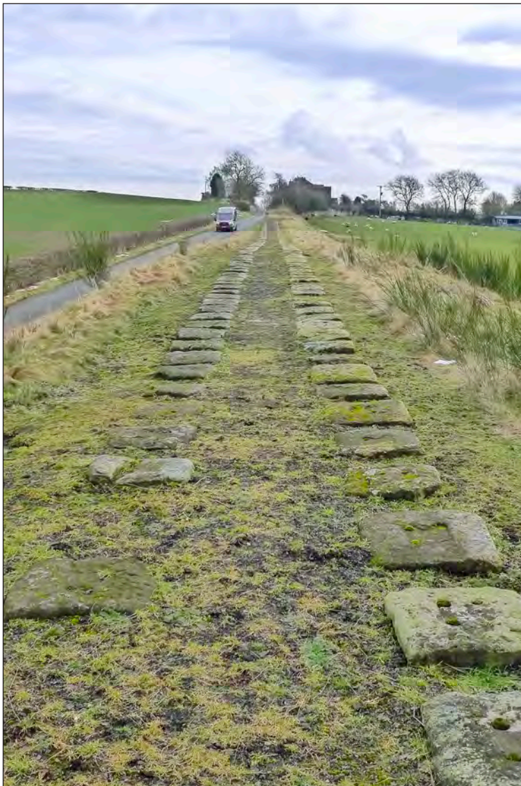
Fig 18: Original stone sleepers from the 1825 railway along the Brusselton West Incline. March 2019 © Historic England.
