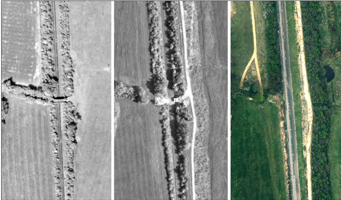
Fig 24: The bridge adjacent to Moordale Park (AIM63) was intact in the 1980s (left). By the mid-1990s, the decking had been removed (middle), but the stonework abutments were intact. The entire structure was then demolished in around 2014 in connection with track improvements (right). Detail of OS/89263 V 39 11-JUN-1989; Detail of OS/93209 V 77 06-JUN-1993 © Crown copyright. Ordnance Survey; Detail of NZ2721 06-MAY-2016 © Bluesky International/Getmapping PLC.
