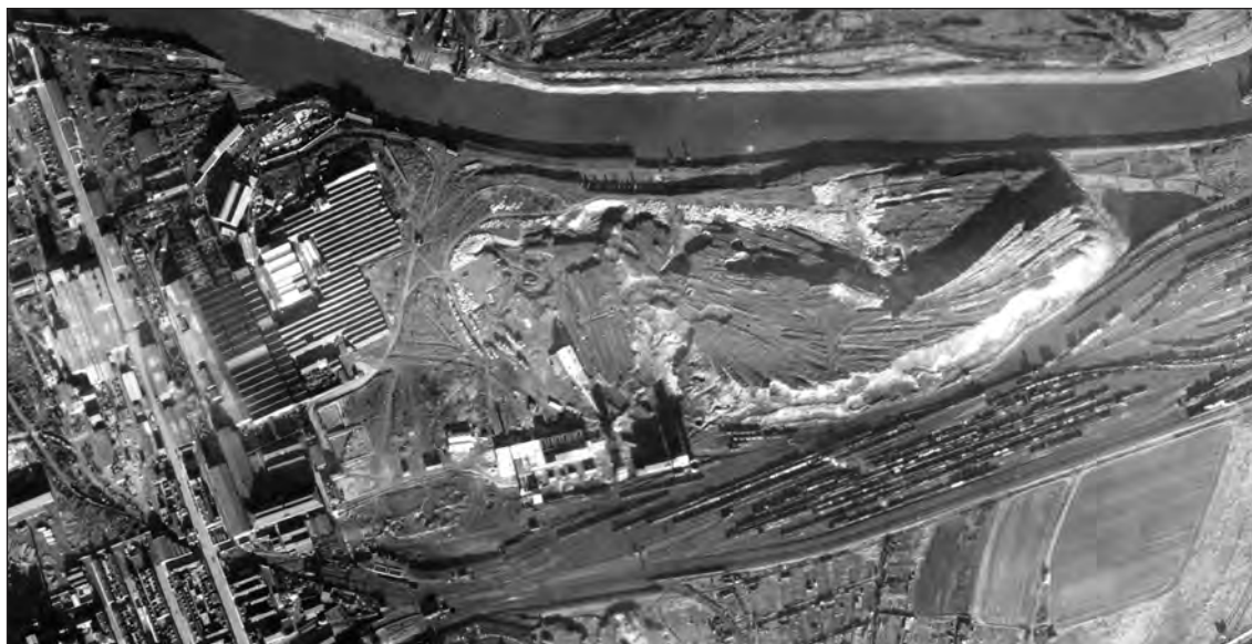
Fig 67: The Thornaby Iron Works (NRHE 1623941) was just one of many situated along the River Tees. In common with many other industries along the S&DR (and later extensions/incorporations), it linked directly into the railway. Detail of RAF/CPE/UK/1835 RS 4213 13-NOV-1946 Historic England Archive (RAF Photography).
