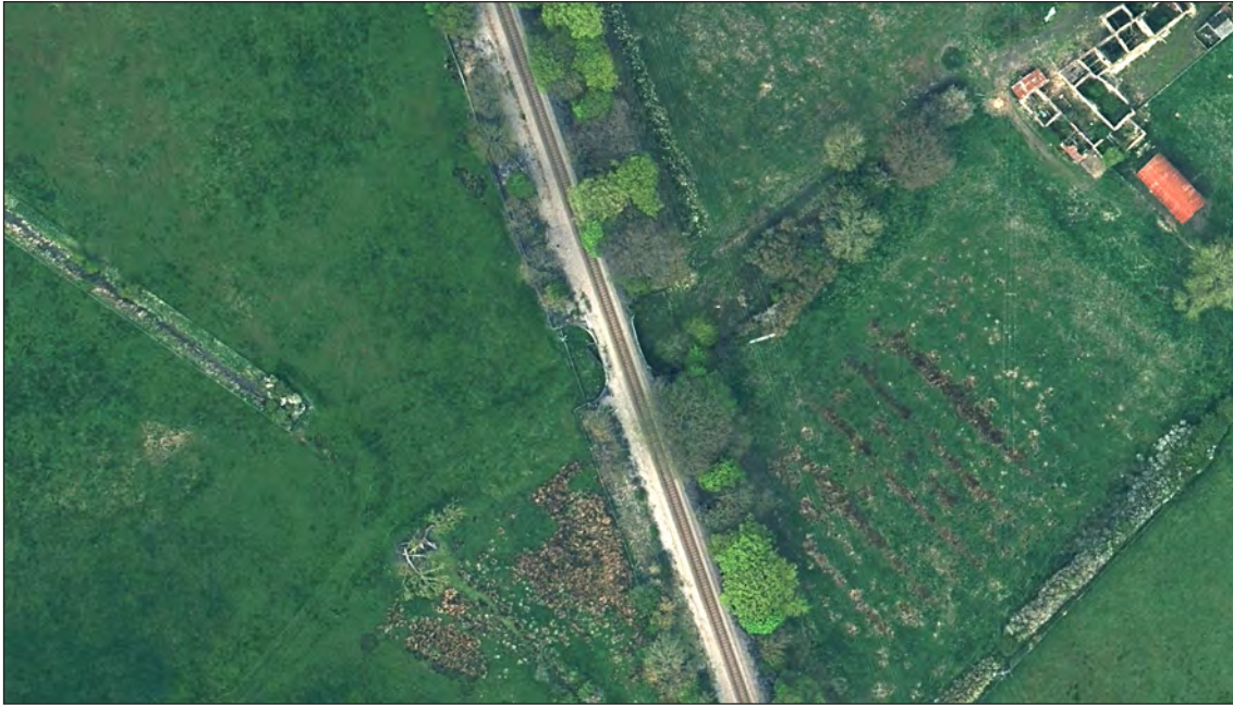
Fig 26: The underbridge that served access to Coatham Grange/Myers Flat (seen in ruins to the right) retains its original curved abutments, though the decking has been replaced (AIM70; HEA194). Detail of NZ2719 06-MAY-2016 © Bluesky International/Getmapping PLC.
