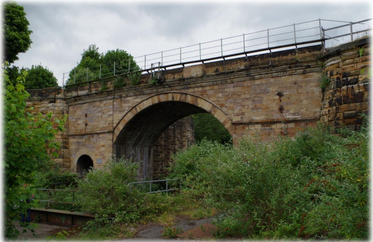
Plate 6. Skerne Bridge today
