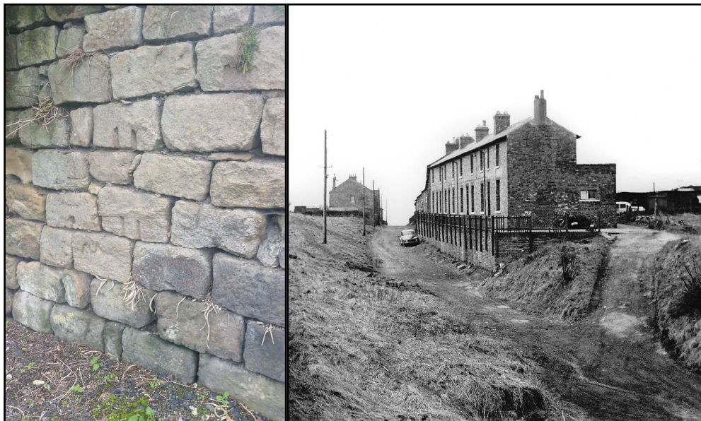
Left: Reused split sleeper blocks
