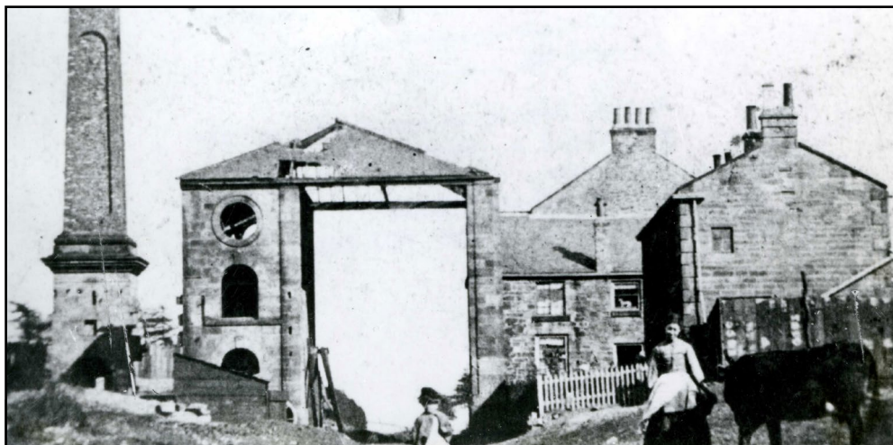
Brusselton Engine House; chimney and winding house now demolished (undated, but possibly c.1880). The large empty building of 1831 held the winding gear which consisted of large drums which sat above the line, powered by the steam engine adjacent. This was a replacement of the first Engine House which still partially survives on site today as a domestic house (to the right).
