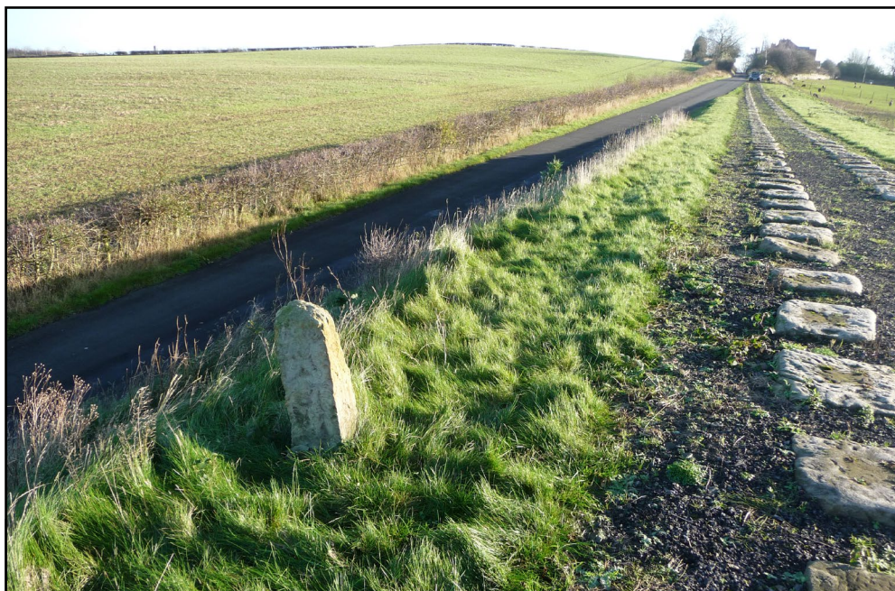
The Brusselton Incline with extant sleepers and an S&DR milestone
