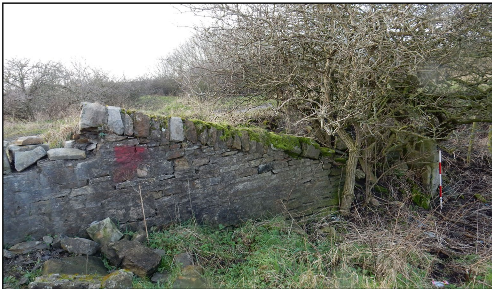
Sloping boundary walls adjacent to a now-buried tunnel. The boundary walls along this stretch of line were all topped with triangular cope stones.
