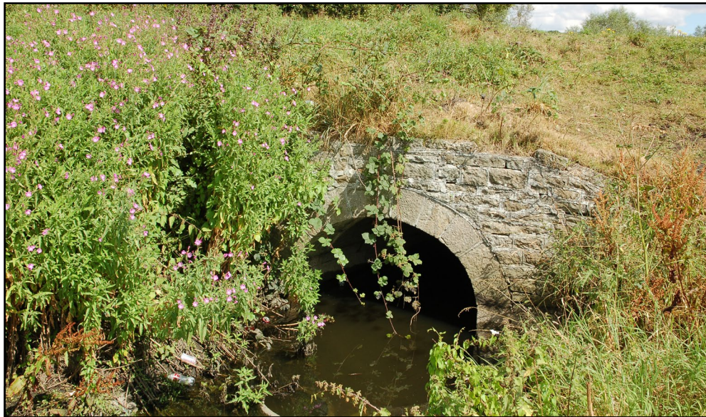
Original 1825 culvert south of West Auckland viewed from below the railway embankment.
