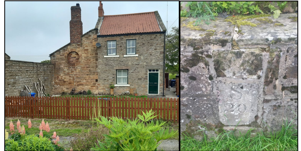
The remains of the engine house and an S&DR milestone, rebuilt into the garden wall.
