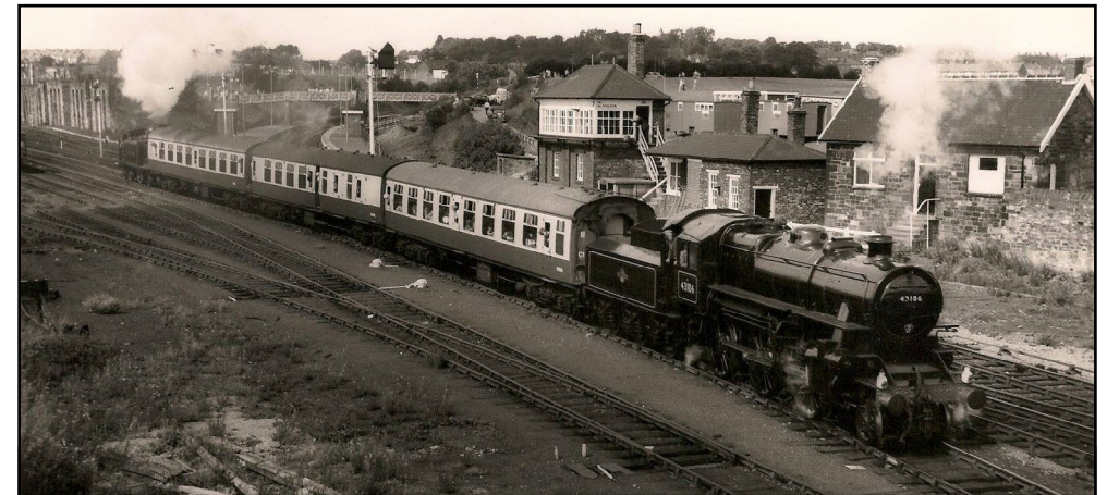
An undated photograph of the signal box and adjacent buildings and the coal drops in the distance. 43106 was built at Darlington in 1951. Although it was originally withdrawn from service in 1968, it is still operational on the Severn Valley Railway
