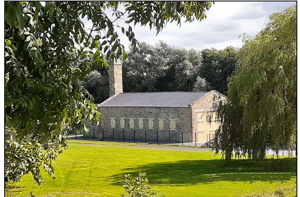
Kilburn's Warehouse. Photo: Ben Goundry
