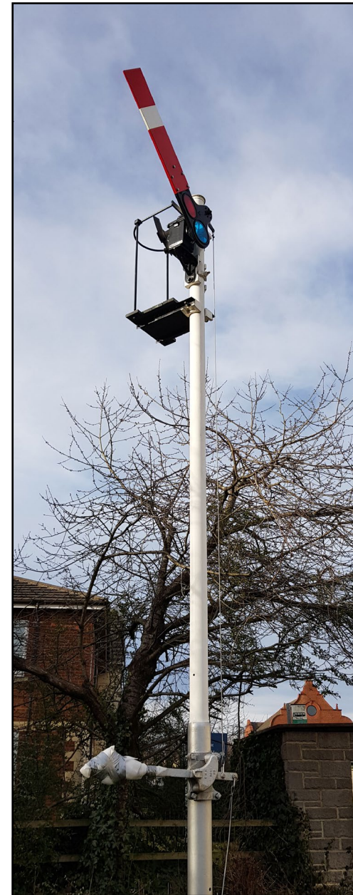
The railway semaphore signal opposite the former Masons Arms. The S&DR Works were located just beyond it.
