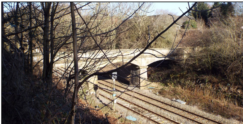
The aqueduct over the Tunnel Branch. Photo: Peter Bainbridge
