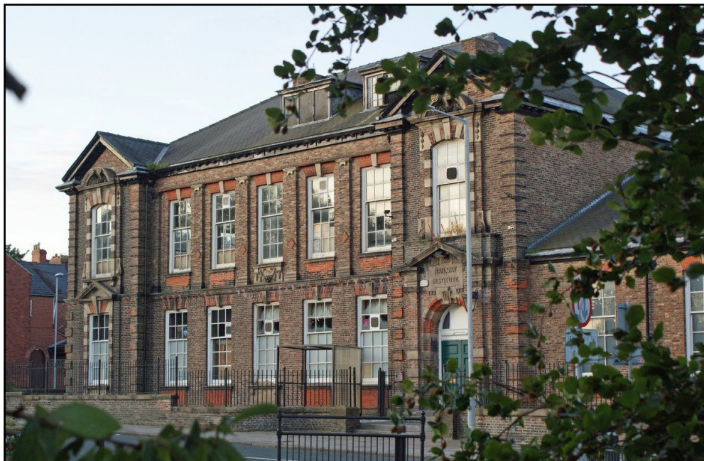
Railway Institute (photo: Dave Reynolds)
