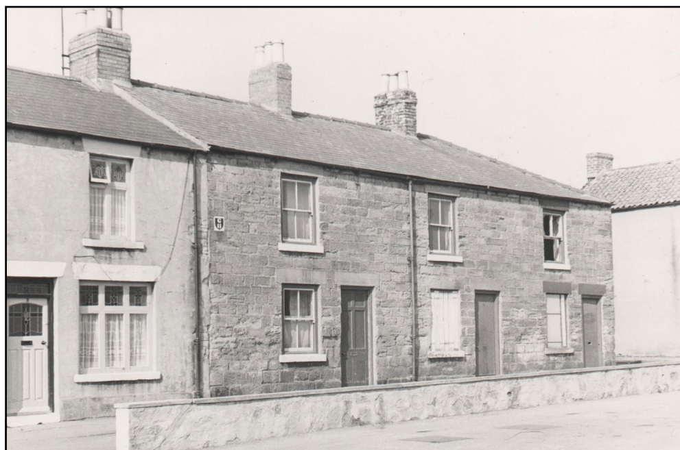
G11 Fulton Terrace in April 1968. This was housing for S&DR workers operating the Black Boy branch and incline, now destroyed and replaced with the doctor's surgery © R Goad with permission
