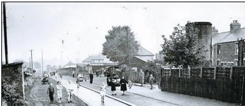
The ventilator shaft (on the right behind the tree) behind Windsor Terrace in 1962 adjacent to the footpath.
