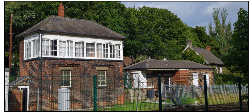
The 1887 signal box, signalman's cottage and possible weigh house to the right.
