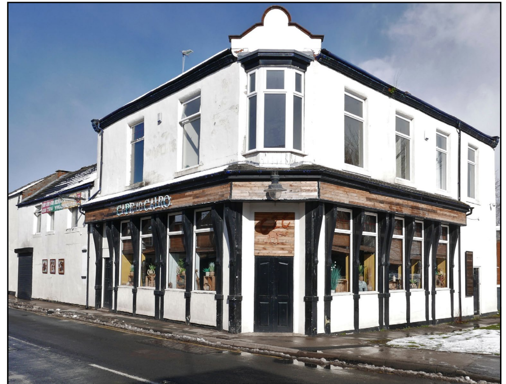
The former Masons Arms (since renamed Cape to Cairo) and site of the Masons Arms Crossing
