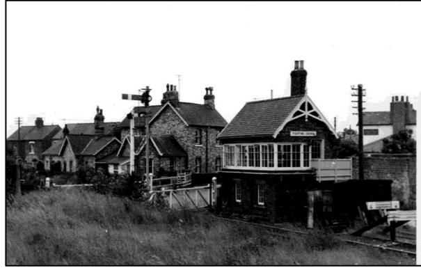
17. General view of the former crossing
