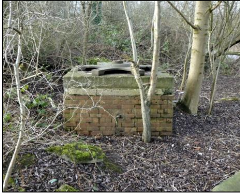
16. The crane base
